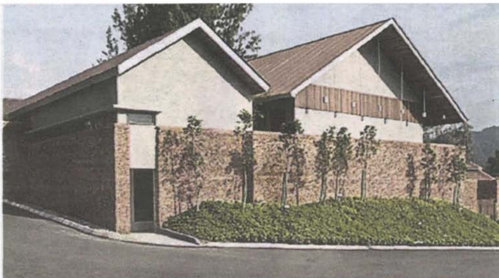
Among the sustainable features are the 'huruvara' brick walls constructed from recycled bricks salvaged from existing buildings on site.
